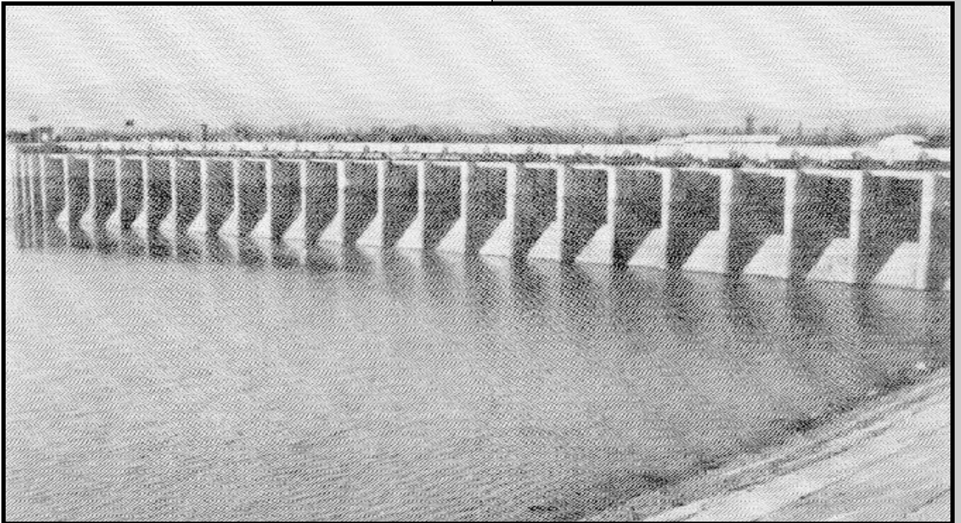
Battery of DCC 2 distributors. Max. flow 114 m 3 /s.
